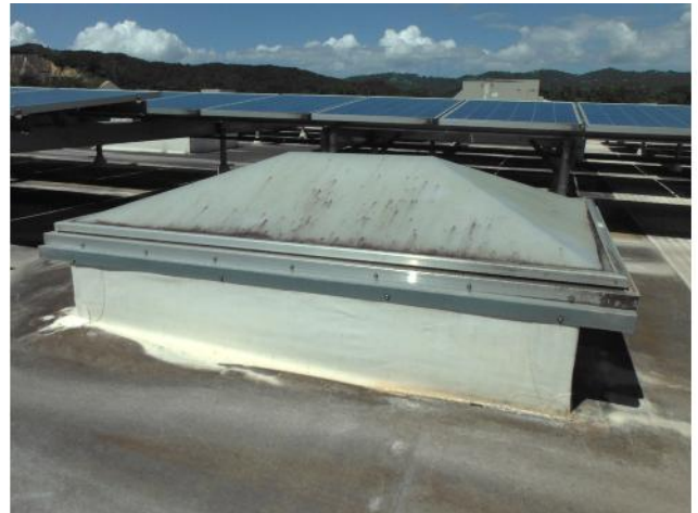
Photo of incorrectly measured custom skylight
